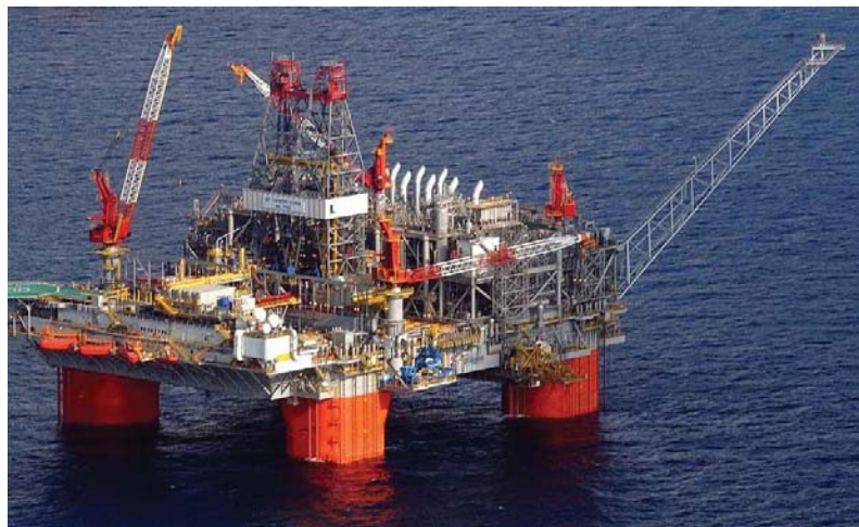
Thunder Horse PDQ deepwater semi-submersible oil platform in the Gulf of Mexico, a joint venture by BP and ExxonMobil. Photo: Andyminicooper / Wikimedia Commons
