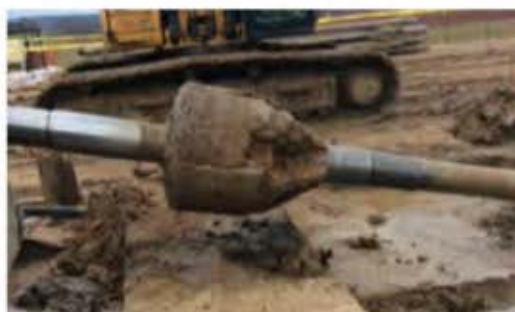
Balled Up Reamer April 3, 2017
