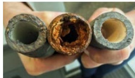
Lead service lines showing inner surface without any coating from corrosion-control treatment (left), with coating (right), and fully corroded (middle). (EPA photo)
