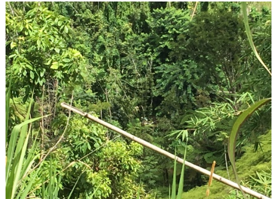
Aboveground drinking water distribution pipe in rural Puerto Rico broken as a result of a hurricane. (EPA OIG Photo)
